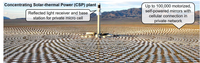
Fig. 1: Concentrating Solar-thermal Power plant as an example for highly dense private NB-IoT networks. Image based on [3]
