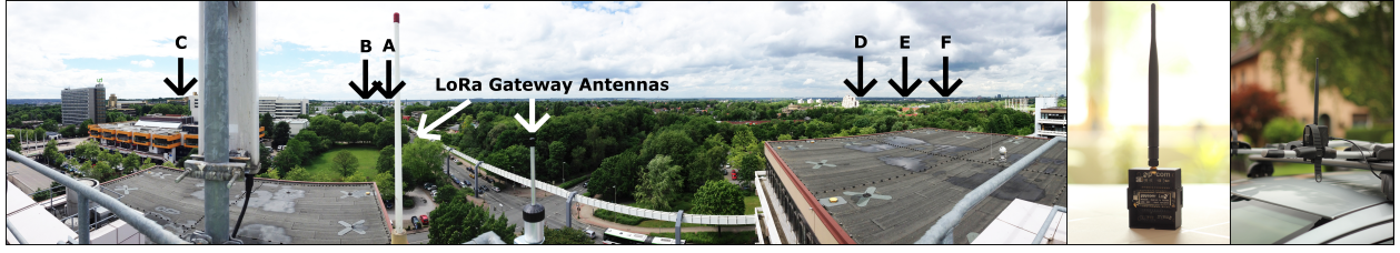
Fig. 1: Installation site of Smart City LoRa Gateway antennas in 30 m height and fixed LoRa nodes A to F (left) as well as Pycom LoRa measurement node (middle) mounted on car (right).
